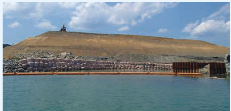
Reconstruction projects (Shizugawa Bay, Miyagi Pref., Jul., 2015)
